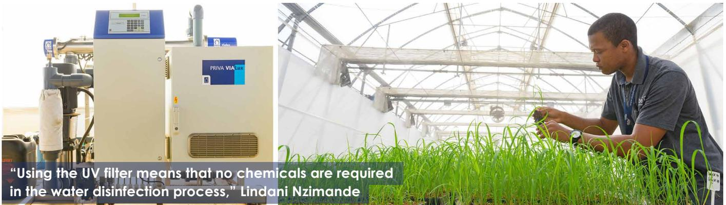
“Using the UV filter means that no chemicals are required in the water disinfection process,” Lindani Nzimande
